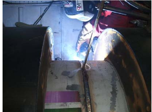
Gas shielded flux cored arc welding, Supercore 308LCF, being used for the first time during construction of the Grain-LNG importation facility on the Isle of Grain, UK. Photograph courtesy of P M Associates UK Ltd.
